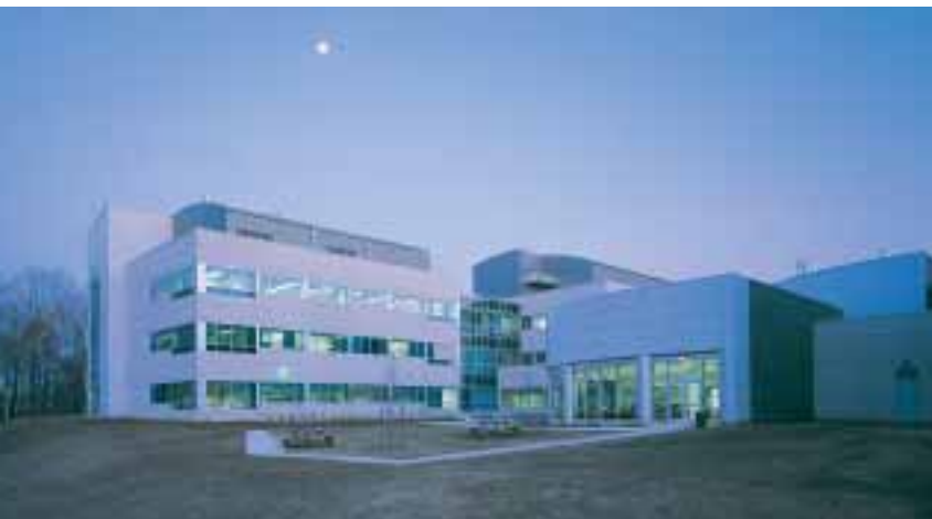
QIAGEN's North American Headquarters, Germantown, Maryland, USA.
